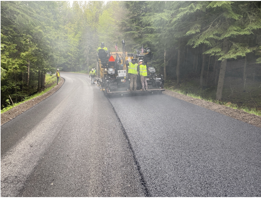
Road Paving Top lift along the GTSR
