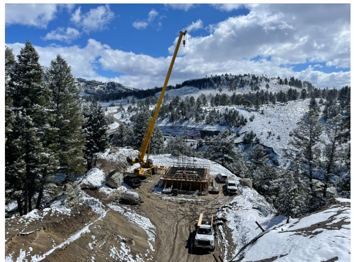
Rebar and Forms at Pier 1 Footing
