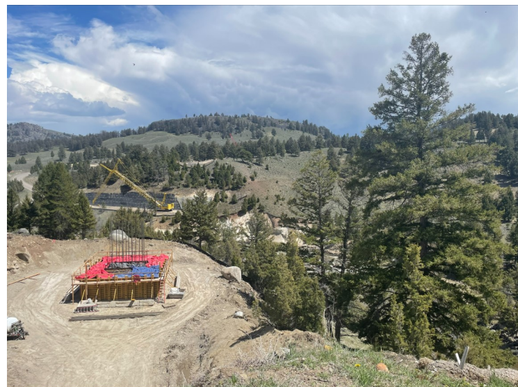
View Down New Alignment
