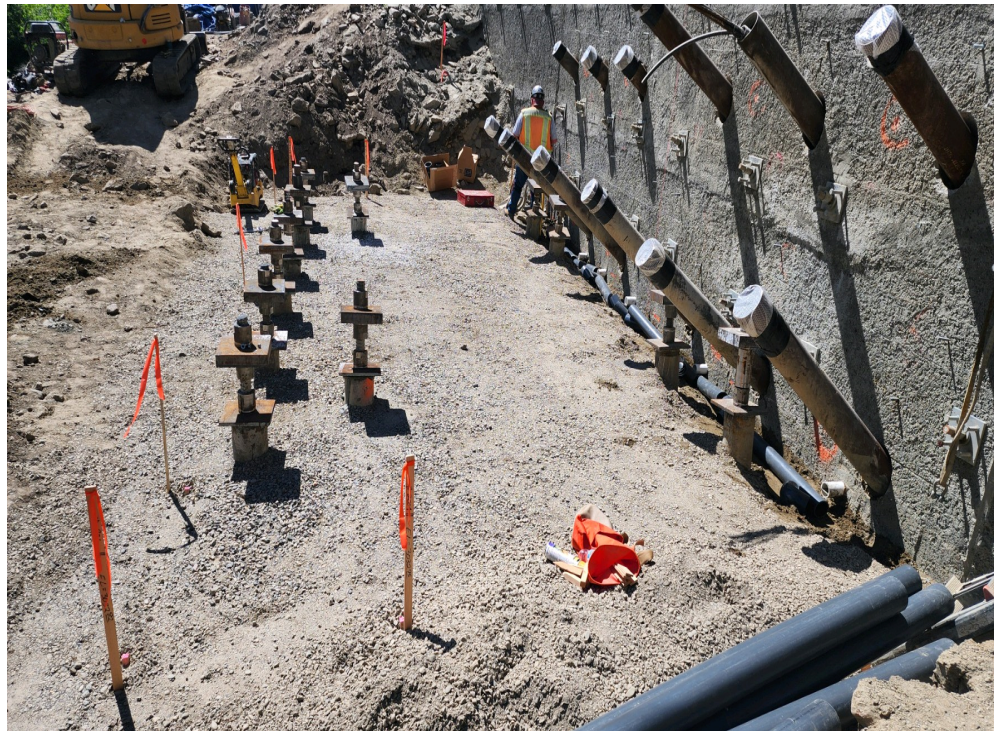
Completed Micropiles
