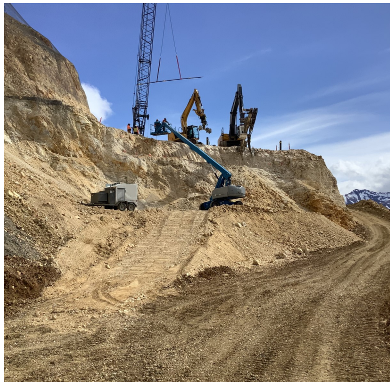
Drilling and installing soil nails at the east abutment.
