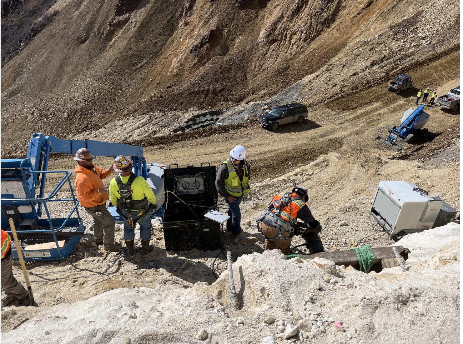
Preparing to proof test a soil nail.
