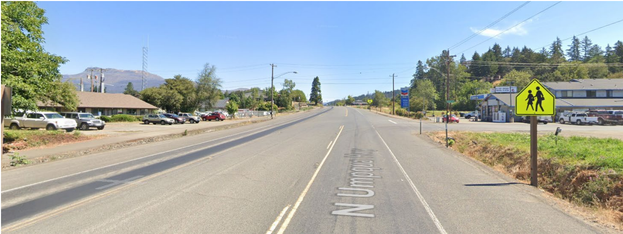
Figure 4. Example of Tier 3 bicycle path (shoulder) from Glide, Oregon. Source: Google Maps 2024.
