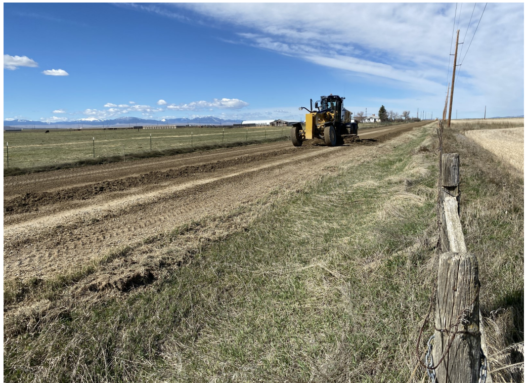
Source: FHWA Reconditioning work along Lower Denton Road
