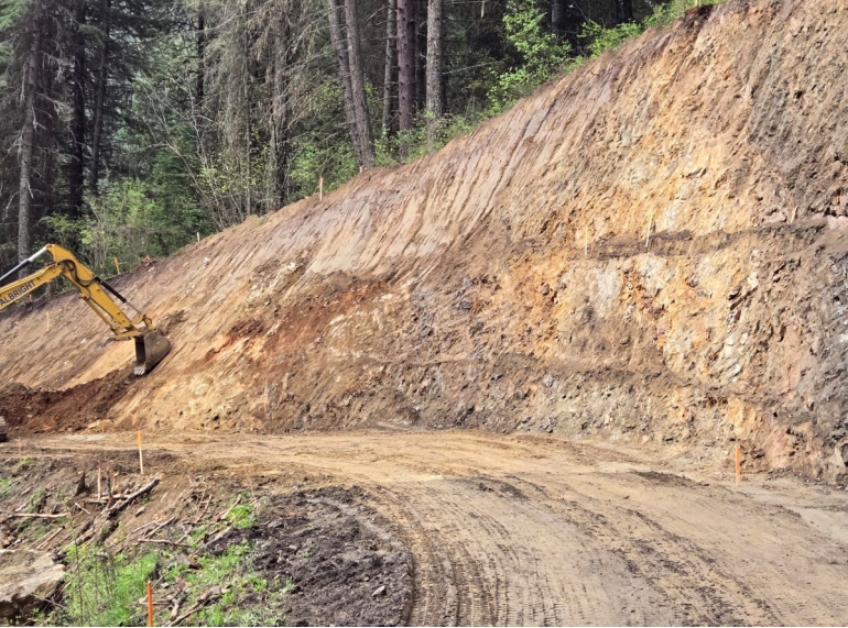
Roadwy Excavation M.P. 13.6 FSR354
