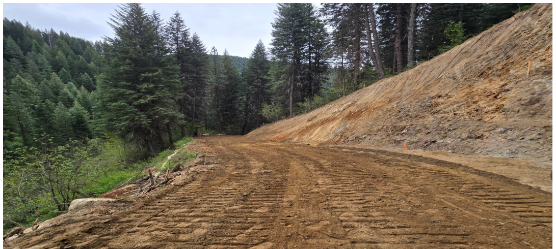
Road bed shaping, M.P. 13.6, FSR354
