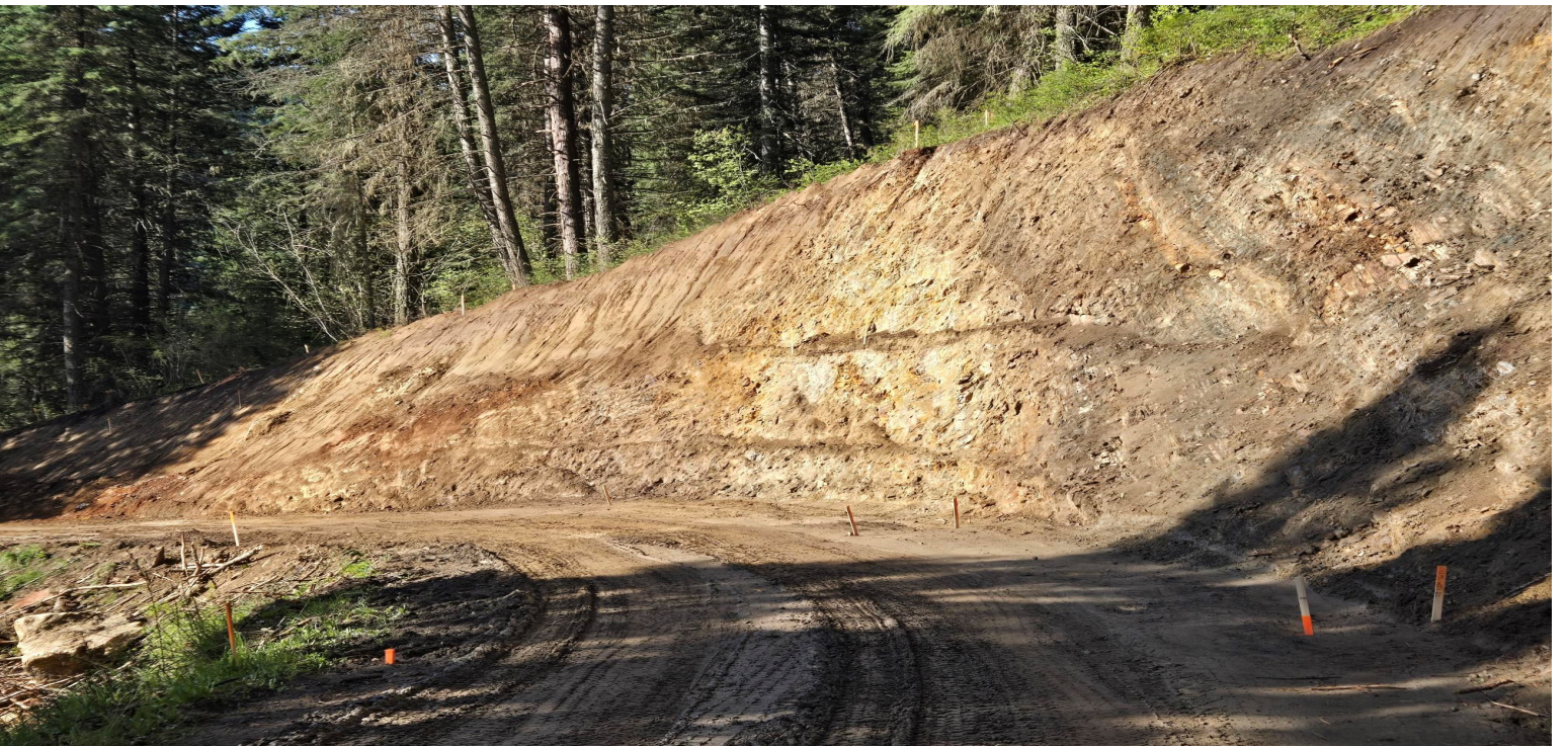
Roadway Excavation at M.P. 13.6
