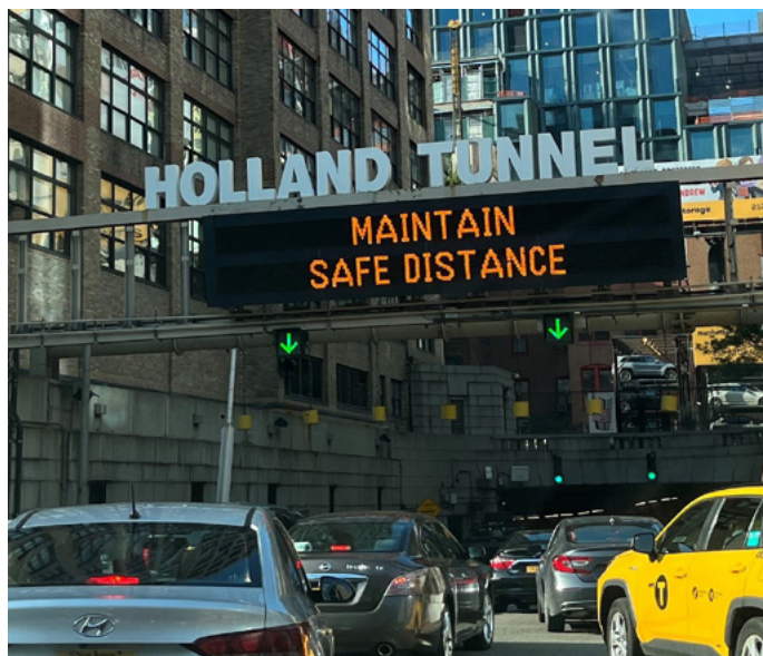
Safety Message at New York Entrance to Holland Tunnel. Photo courtesy of PANYNJ.
