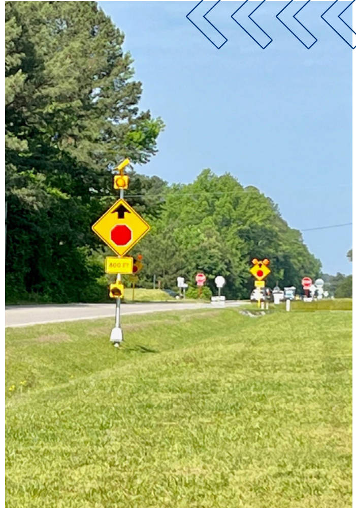
Series of Advance Signage approaching an All-Way Stop in NC. Photo courtesy of NCDOT.
