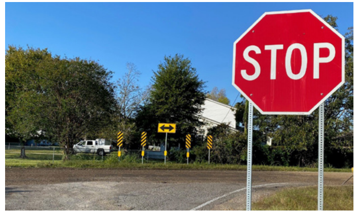
Oversized Stop Sign with Double Arrow Sign and four Object Markers to delineate a T-Intersection. Photo courtesy of Ashley Moran, Acadiana Planning Commission.
