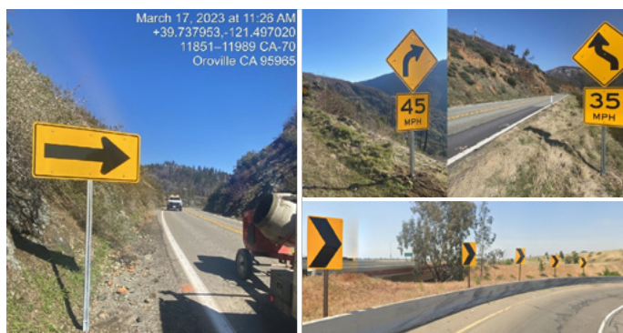
Horizontal Curve Warning Sign Packages. Advance Curve Warning with advisory speed limit sign, chevron, and arrow signs. Photos courtesy of Caltrans.
