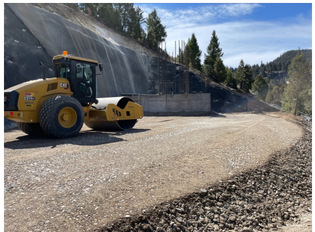
Crane Pad and Backfill Pier 3
