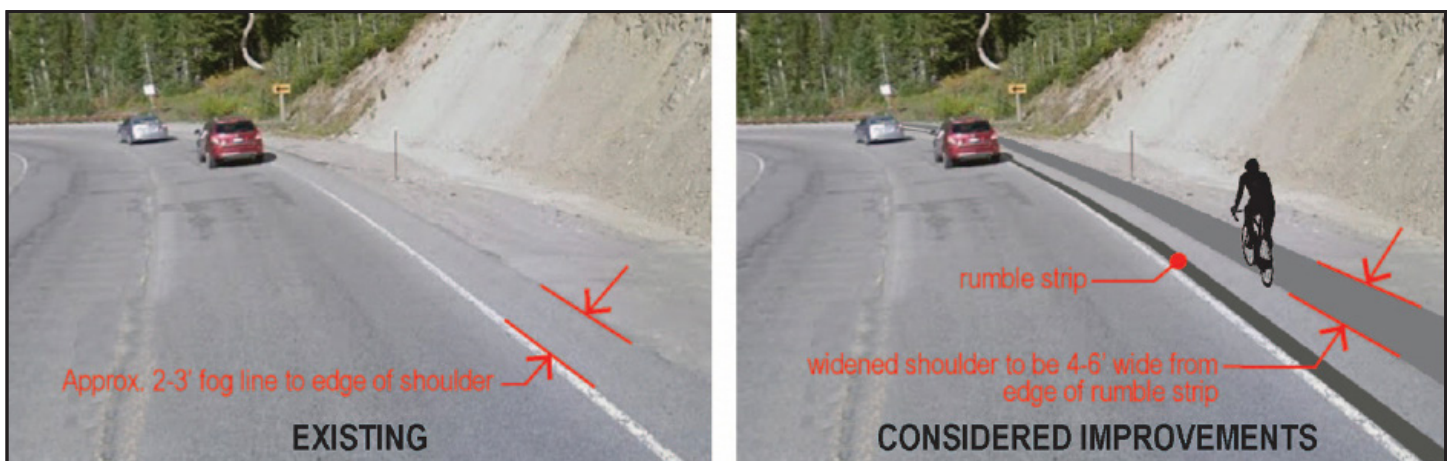
Figure 44: WY-22 Milepost 12.7 existing and considered improved shoulder treatments
