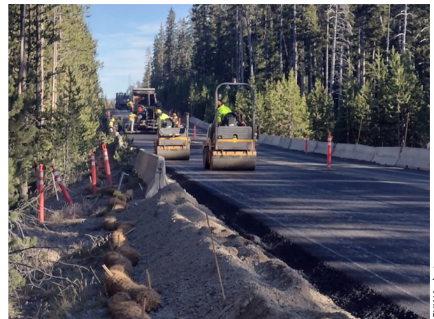
Above: Temporary paving has been placed over all sub-excavations on the Grand Loop. Temporary guard rail, and erosion control measures are in place.
