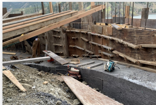
Retaining Wall Form Work in West Portal Overlook
