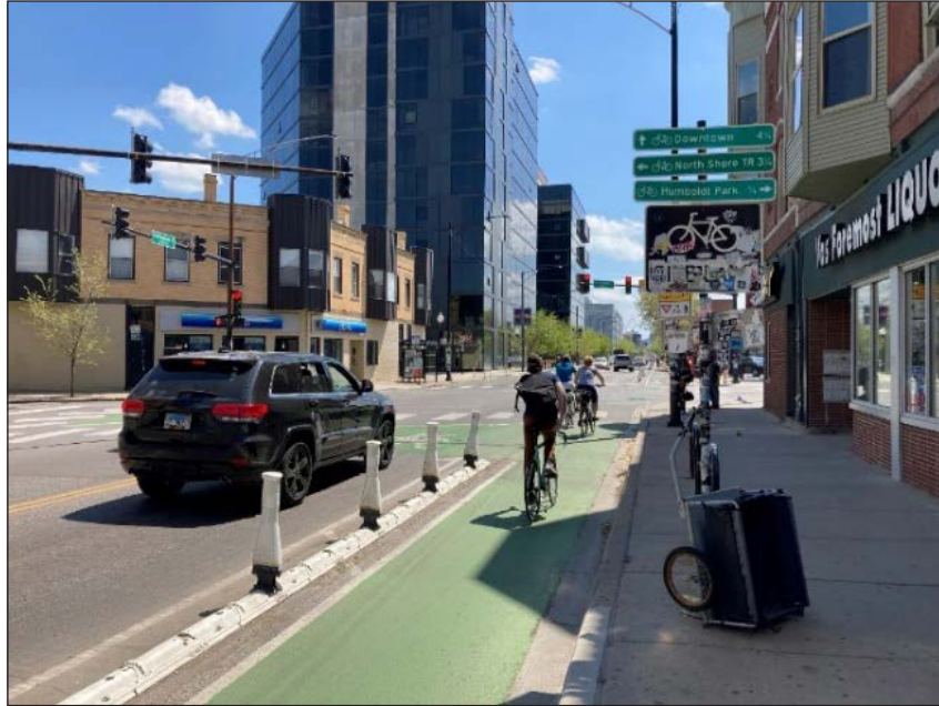
Figure 3. Image. Plastic curbs and green bike boxes at the Milwaukee Avenue and California Avenue intersection.
