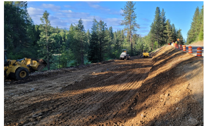
Embankment construction
