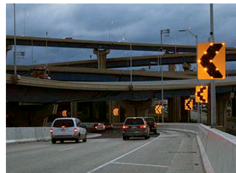
Figure 3. Example of sequential dynamic curve warning system.
