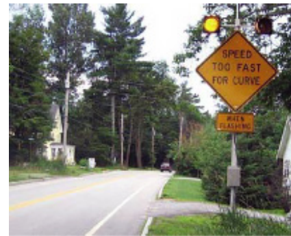
Figure 2. Flashing beacon with warning sign.
