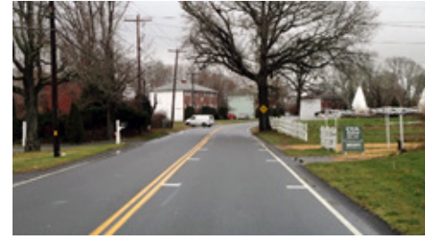
Figure 4. Optical speed bars.
