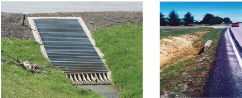
Figure 13. Photograph. Roadside culvert and treatment and associated ditch improvement. 6
