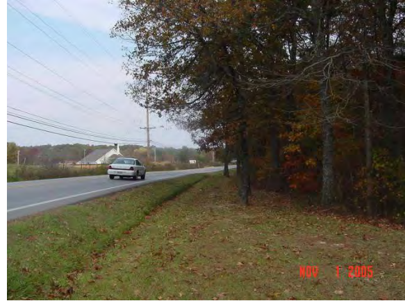
Limited sight distance looking north at L.M. 20.81.
