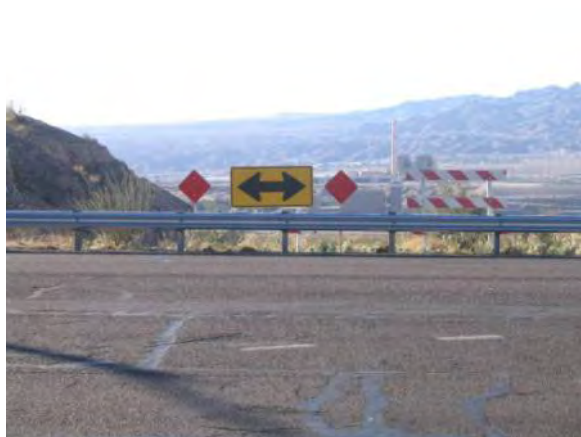
Enhanced T-intersection signing.
