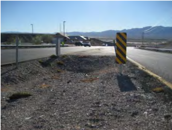
Nontraversable median drains.
