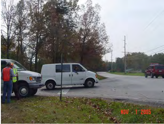
Limited sight distance looking south at L.M. 20.81.
