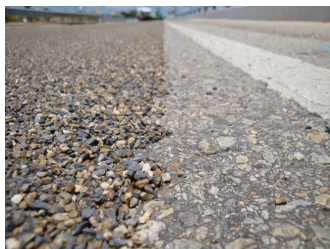
HFST installed on pavement. (Source: The Transtec Group, Inc.)
