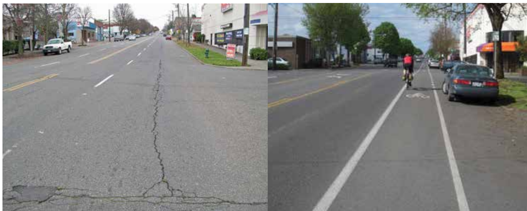
Before (left) and after (right) pictures of Stone Way North. (Source: Seattle DOT)
