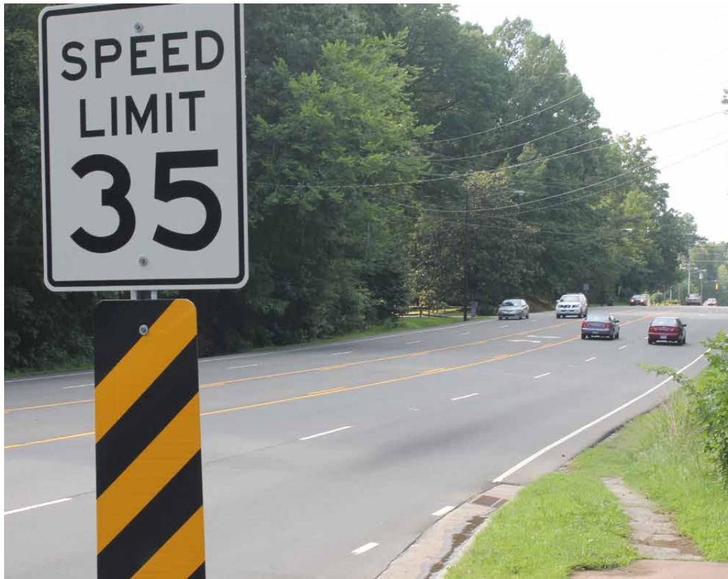
The intended speed of this road is 35 miles per hour, but the wide design of the road and the number of lanes leads drivers to drive much faster.
