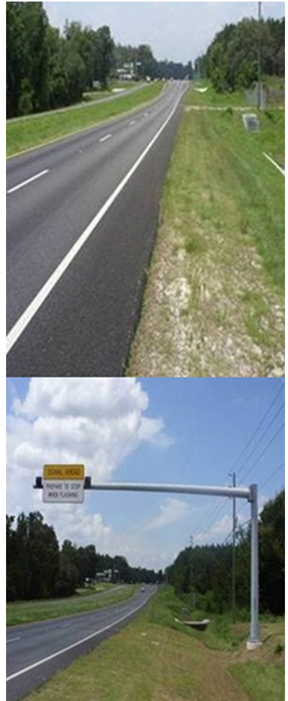
Figure 8-1. Improved Overhead Signage in District 7: Before (top) and After
