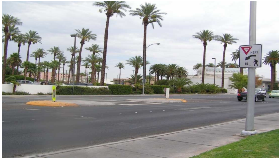
Figure 15: Yield Here to Pedestrians Sign installed at Site 5
