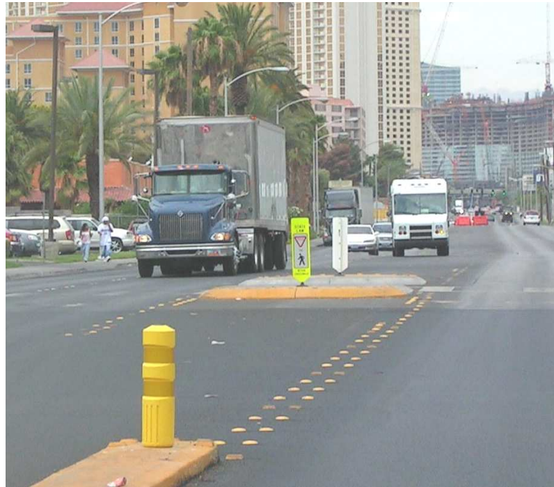
Figure 16: In-roadway Knockdown Signs installed at Site 5
