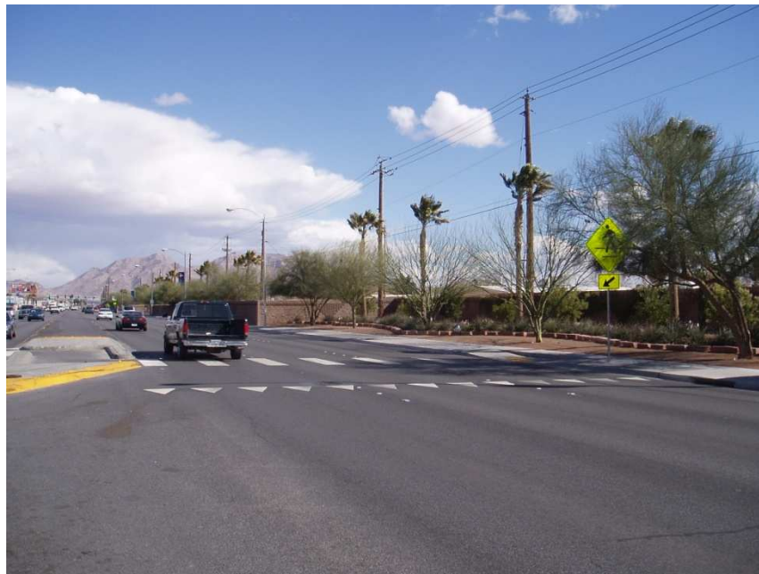
Figure 38: Advanced Yield Markings installed at Lake Mead Boulevard: Belmont Street to McCarran Street
