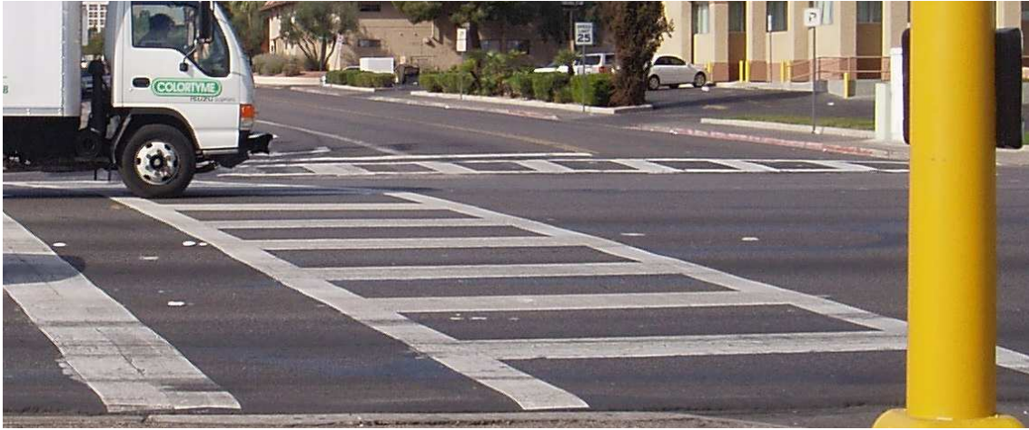
Figure 18: High Visibility Crosswalk Treatment installed at Site 7
