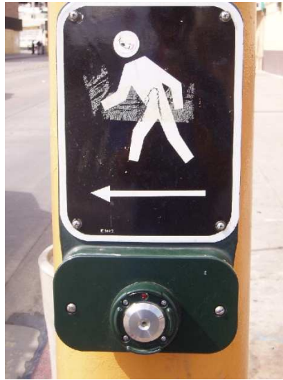
Figure 45: Pedestrian Push Button that Confirm Press
