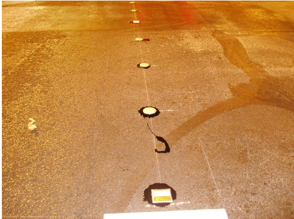
Figure 4. Reflective Pavement Marking (RPM) standard line at Site 1
