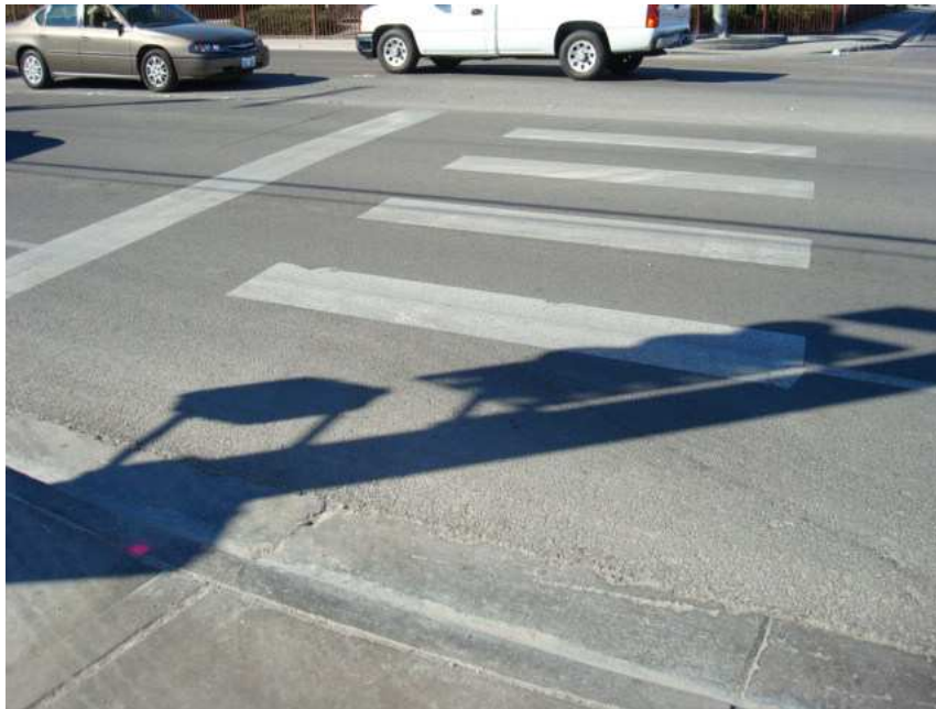
Figure 25: High Visibility Crosswalk Treatment installed at Site 9/10
