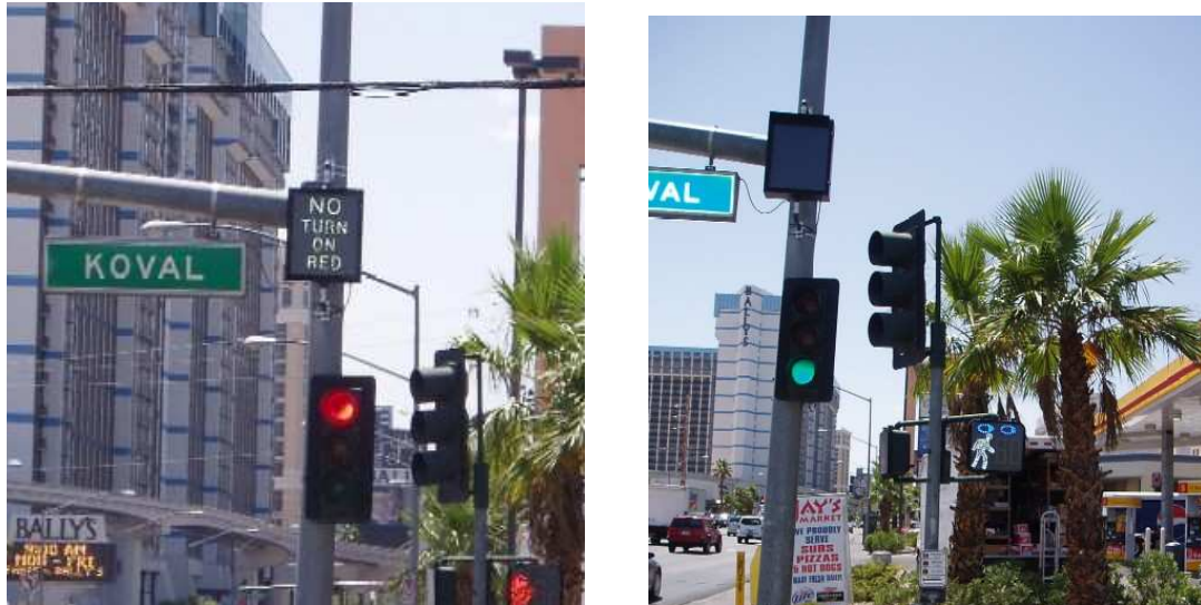
Figure 20: ITS No-Turn On Red – Activated
