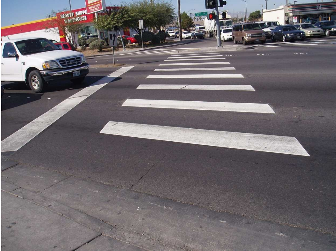
Figure 34: High Visibility Crosswalk Treatment installed at Lake Mead Boulevard and Las Vegas Boulevard
