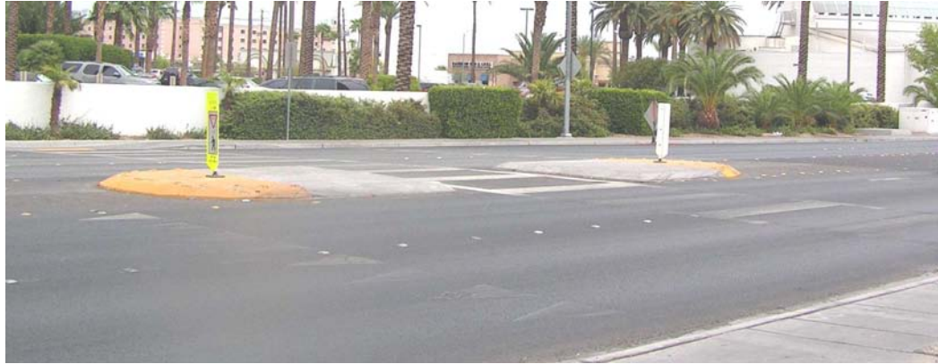
Figure 14: High Visibility Crosswalk and Median Refuge installed at Site 5
