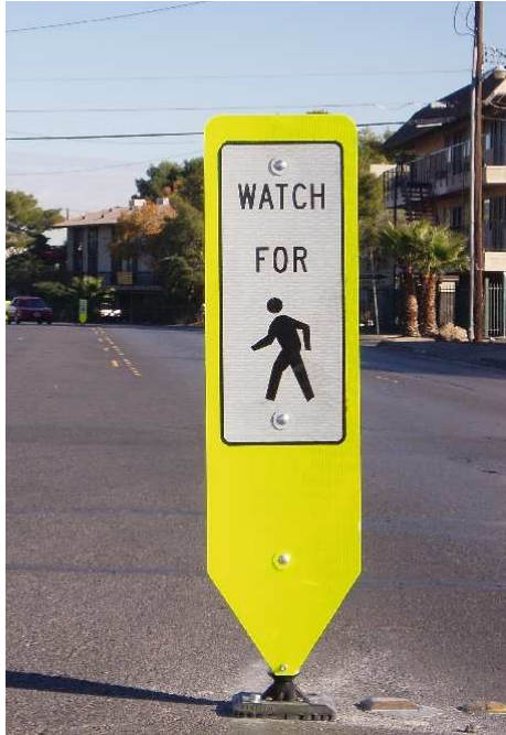
Figure 31: Close-up view of “In-Roadway Knockdown Signs” installed at Sites 11 and 12
