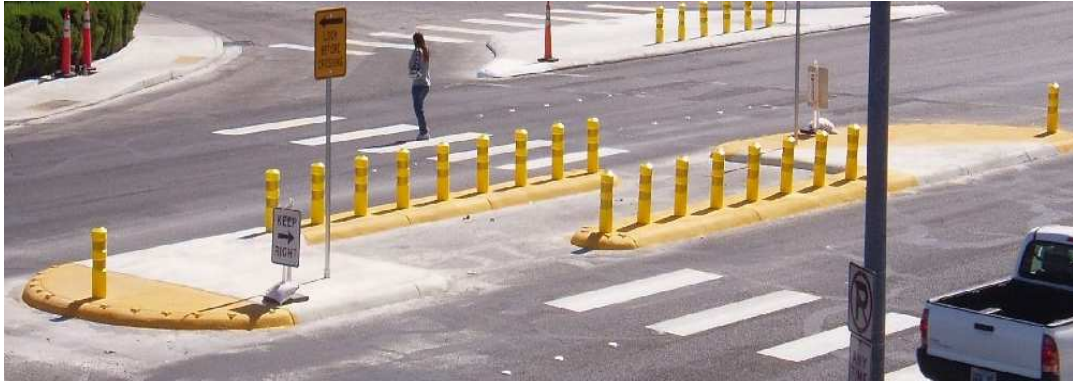
Figure 7: High Visibility Crosswalk Treatment, Median Refuge and Danish Offset
