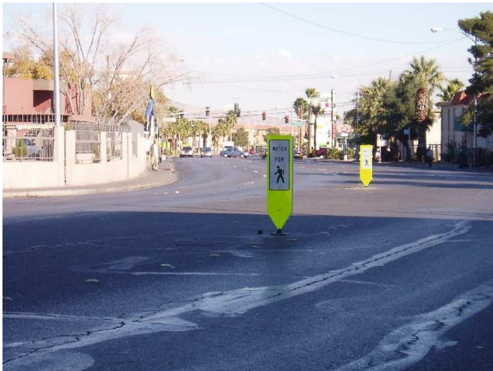
Figure 30: In-Roadway Knockdown Signs installed at Sites 11 and 12
