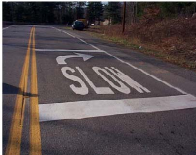
Figure 2. Photo. Horizontal curve warning and speed advisory pavement marking (Retting and Farmer 1998).
