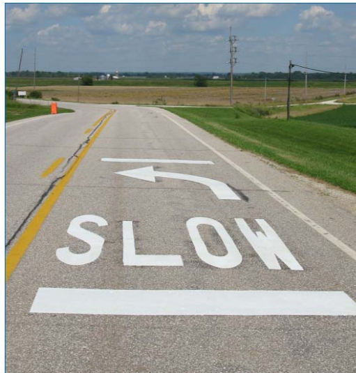
Figure 4. Photo. On-pavement marking (Hallmark et al. 2012).
