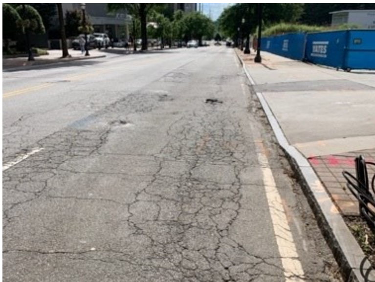
Figure 7. Distressed asphalt pavement.
