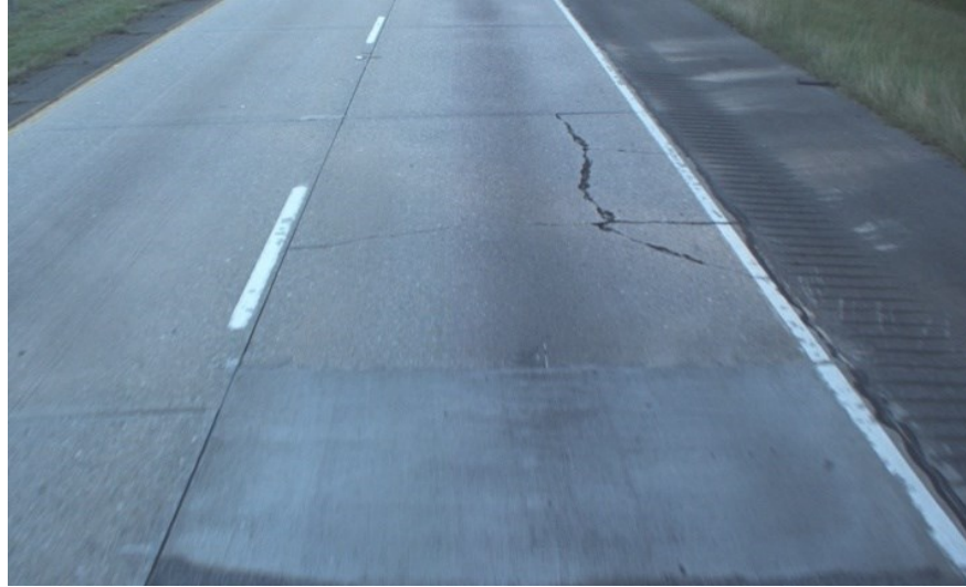
Figure 8. Distressed concrete pavement.
