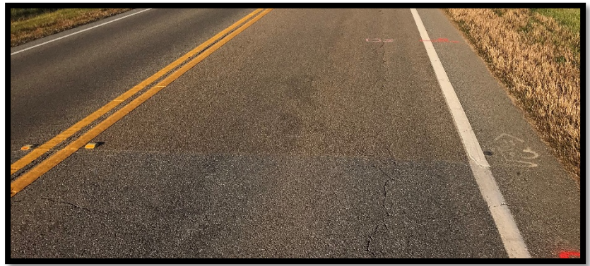
Figure 1: HFST Pavement Treatment Photo Source: Georgia Institute of Technology, March 2020.
