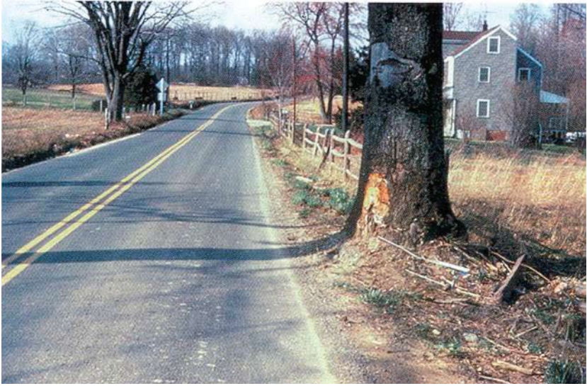
Trees near the road that have been struck before deserve special attention.
