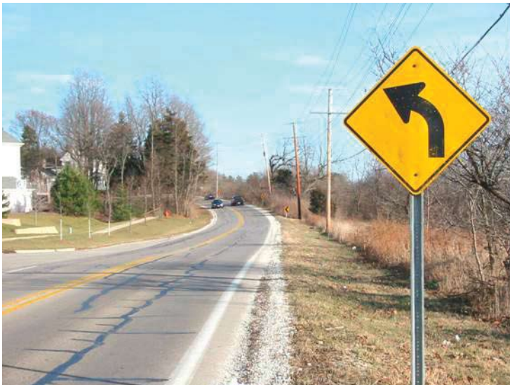
Well-defined shoulder and ditch allow drivers to see the shape, condition, and limits of the roadside.
