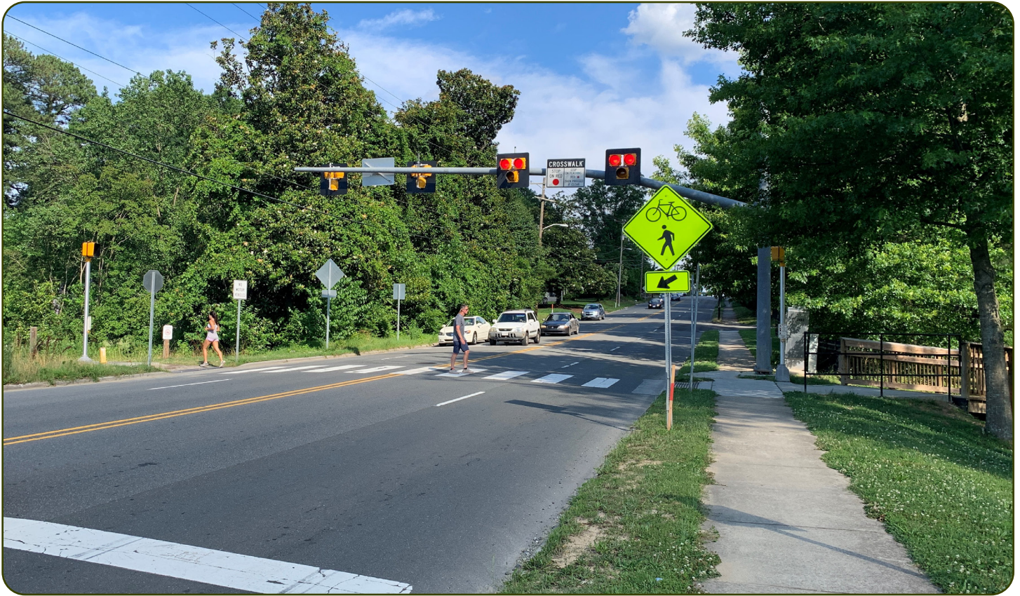
Figure 4: Mid-block trail crossing with PHB. Source: FHWA
