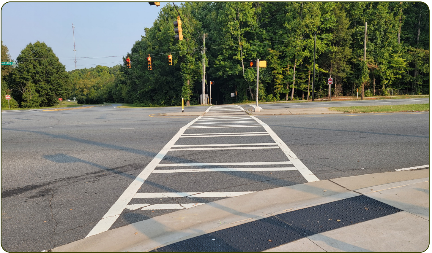
Figure 10: Trail crossing at a complex intersection with a wide refuge. Source: FHWA
