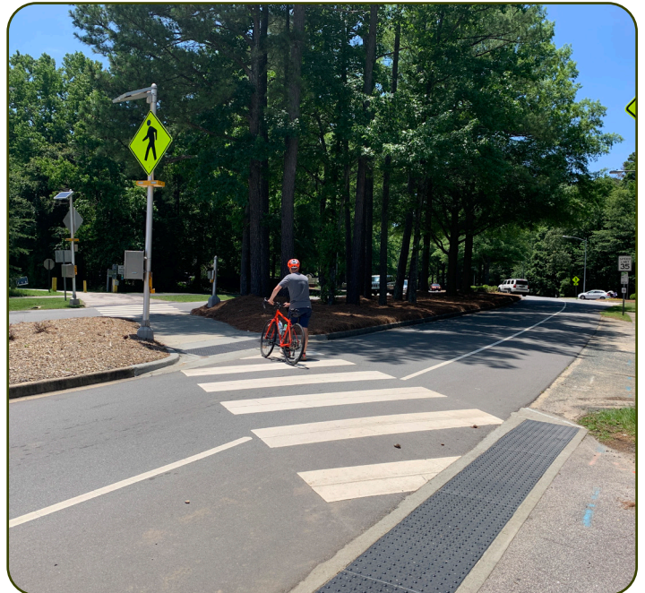
Figure 5: Mid-block trail crossing with RRFB. Source: VHB
