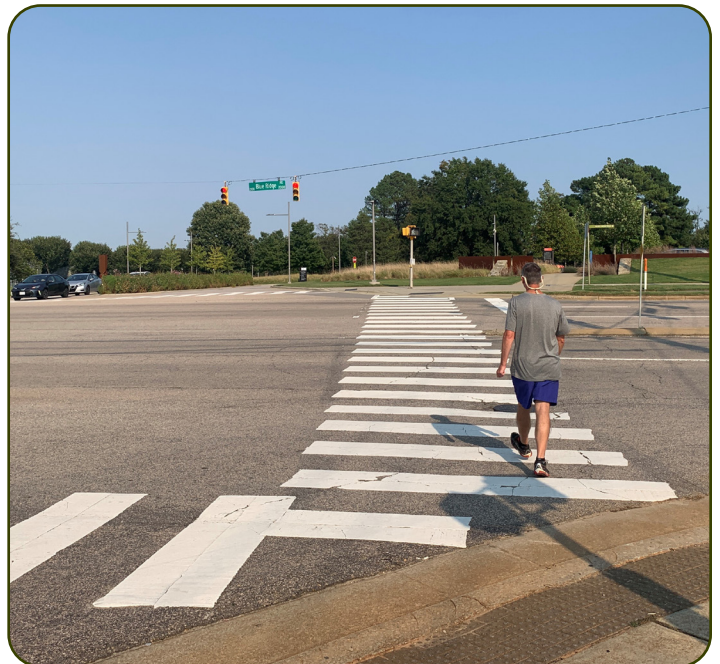
Figure 11: Trail crossing at complex intersection. Source: FHWA
