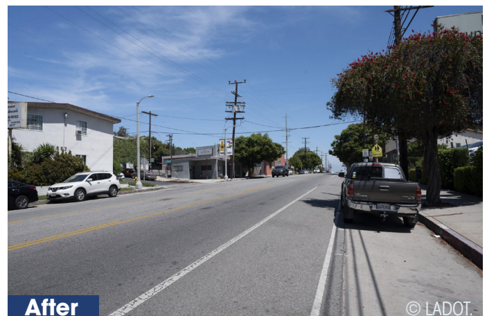
Figure 2. Photo. Rowena Avenue after the road diet with two-way left-turn lane, bicycle lanes and on-street parking.
