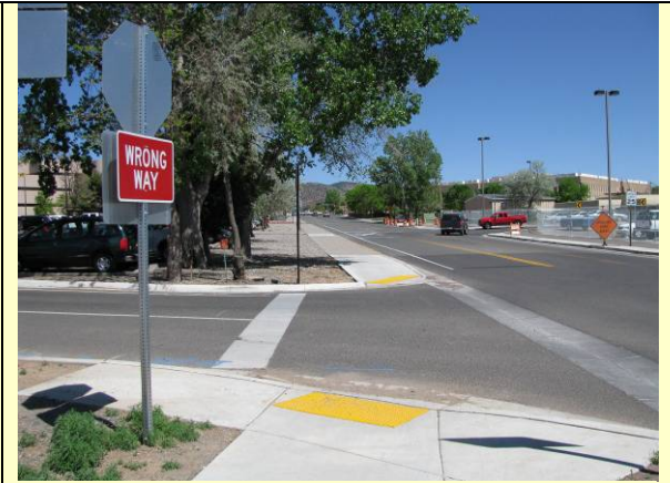
Photo shows curb ramps and truncated domes that are not aligned with the crossing. The ramps and tactile warnings are actually leading people into the adjacent travel lane.
