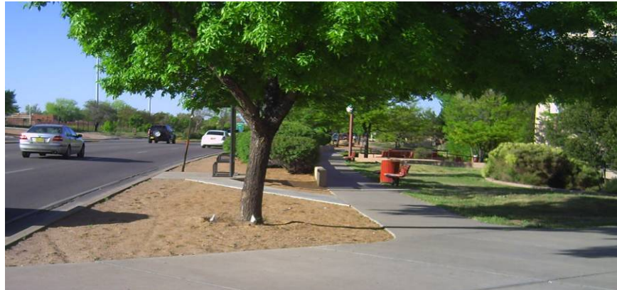
View of southwest quadrant of the intersection of St Francis Drive and Cordova Road. Photo shows where trees and bushes have been planted to provide a buffer strip between the sidewalk and roadway.
