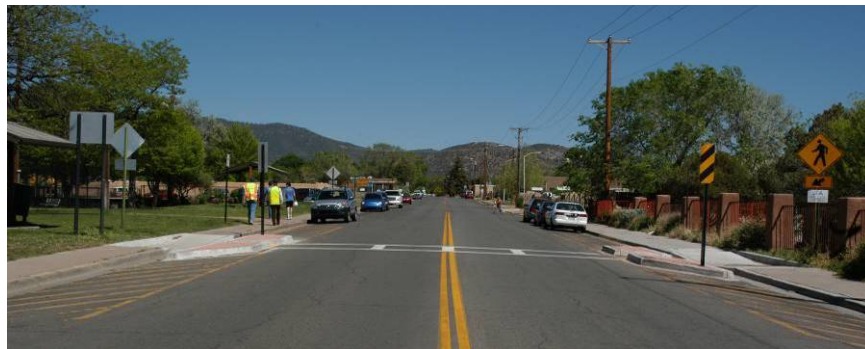
View of Alta Vista Road looking eastbound between St Francis Drive and Luisa Street. Photo shows a neck-down strategy where the pedestrian crossing distance has been reduced by providing raised islands near the edge of the travel lanes.
