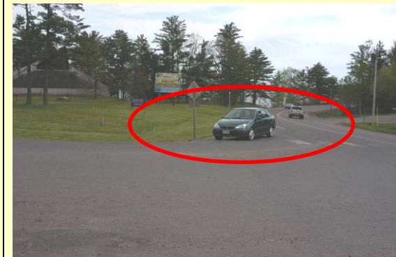
View of intersection of Highway 13 and Blueberry Rd. Photo shows a driver using the shoulder as a right-turn lane. There is a crosswalk at this location and pedestrians are often waiting on the corner.
