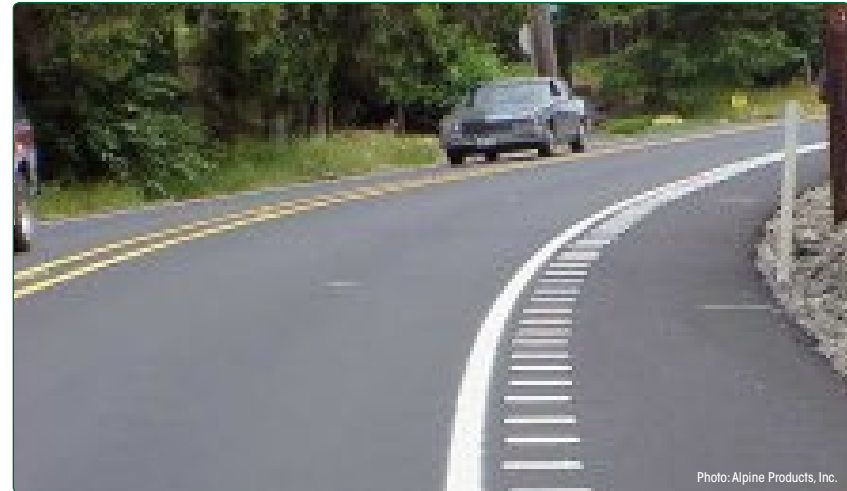
FIGURE 7. Example of Raised Rumble Strips
