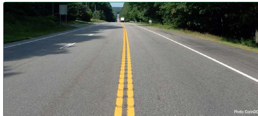
FIGURE 1. Center Line Rumble Strips
