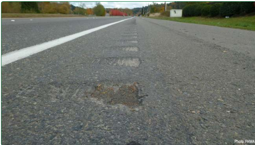
FIGURE 6. Poor Results Due to Differing Cross Slopes
