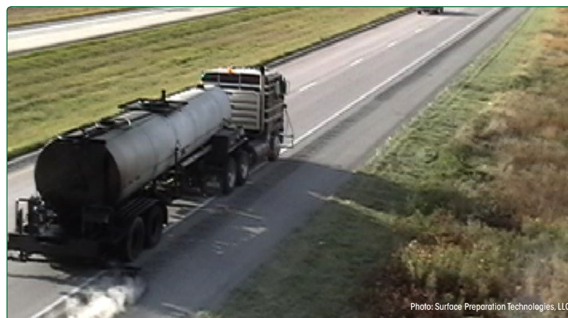
FIGURE 8. Fog Seal Application
