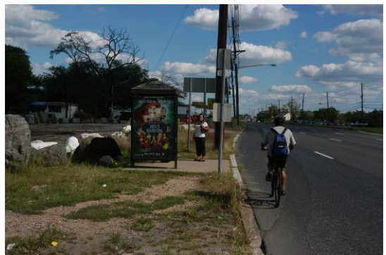
Photo shows the bus shelter along westbound Route 70. The closest crossing of Route 70 is located on the east leg of Cornell Avenue over 2500 feet away. Note also the lack of connectivity between existing sidewalks and the shelter.
