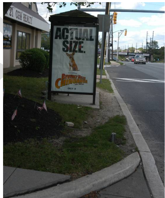
View of bus shelter along Route 70 just east of Garden Park Blvd. Note the lack of connectivity between the existing sidewalks and the shelter.
