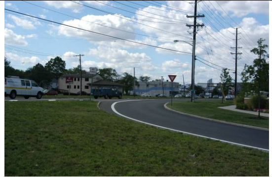
View of channelized right-turn lane on southbound approach at Haddonfield Road. The separator island creates a gap in the connection between sidewalks along either side of the intersection.
