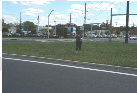
View of channelized right-turn lane and separator island on southbound approach at Haddonfield Road. The RSA team observed pedestrian activity in the area; however, there is no sidewalk or other crossing features in the separator island, resulting in pedestrians crossing at multiple locations.
