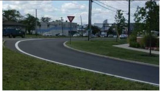
View of channelized right-turn lane on southbound approach at Haddonfield Road. The wide radius allows vehicles to make high-speed turns, which creates a potential safety issue for pedestrians turning to cross the street.
