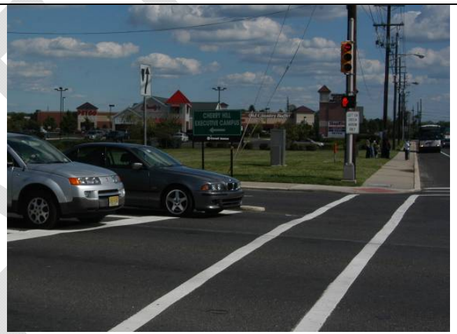
Intersection at Cornell Avenue. Photo illustrates a proper use of crosswalks, curb ramps, and pedestrian signals to enhance safety for pedestrians. The stop bar is also placed before the crosswalk to separate vehicles from pedestrian traffic.
