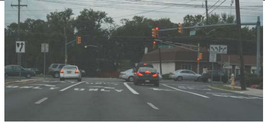
View of southbound approach at Cornell Avenue showing the dual right-turn configuration.
