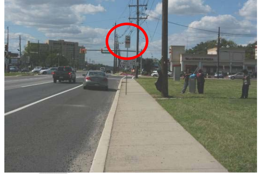
Photo shows the wide shoulder on the westbound approach at Cornell Avenue. As can be seen in the photo, a motorist is using the shoulder as a travel lane. This is a concern because there is a bus stop on this approach (as shown by the red circle).
