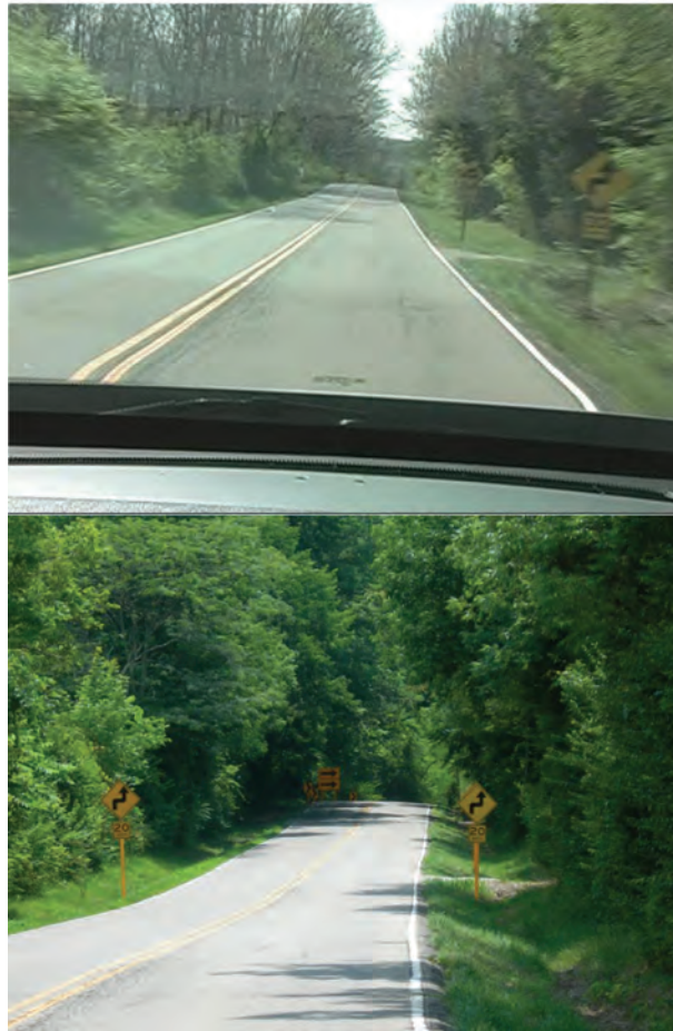
Figure 4.5 Before and After Photos of Sign Installation
