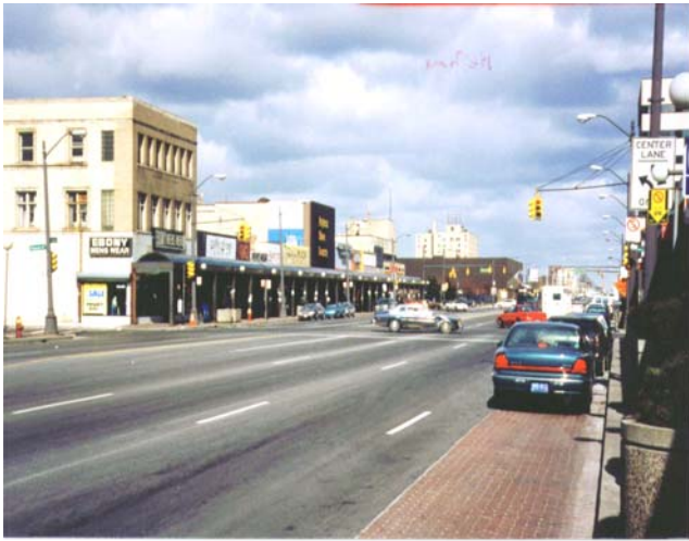
Photograph 1. Woodward Avenue at Milwaukee Street ('Before' Condition)
