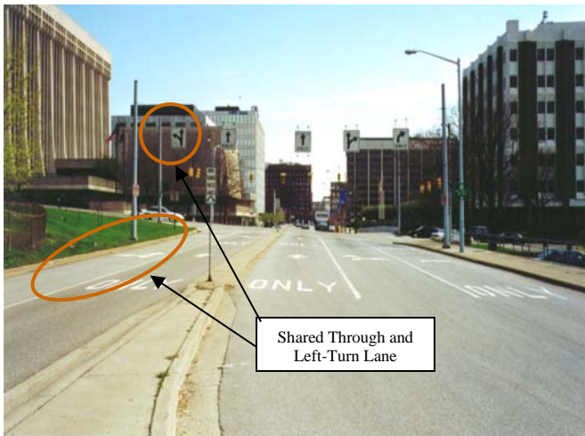
Photograph 27. Southbound Ottawa Avenue at Michigan Street ('Before' Condition)
