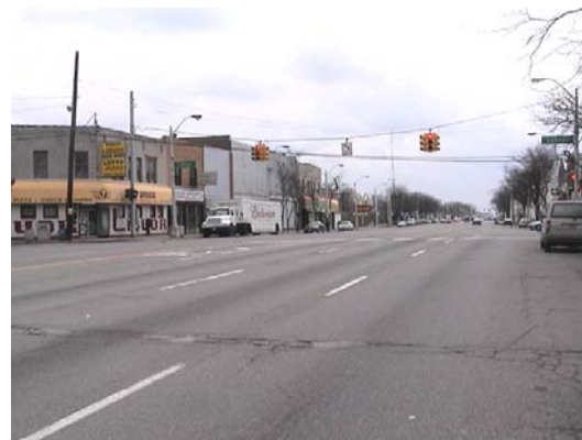
Photograph 8. Grand River Avenue at Lahser Road ('After' Condition)
