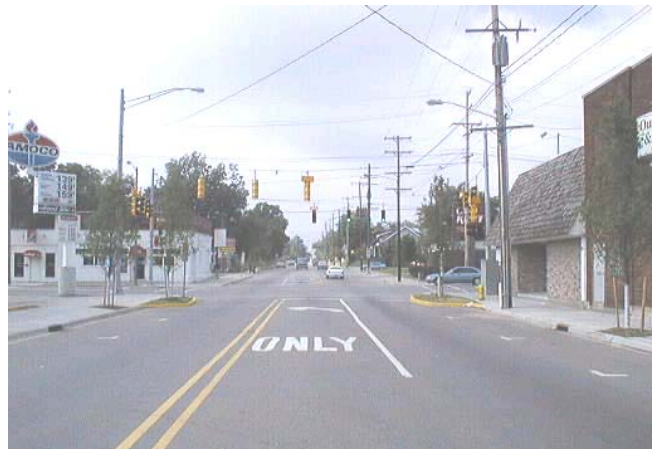
Photograph 18. Eastern Avenue and Franklin Street ('After' Condition)
