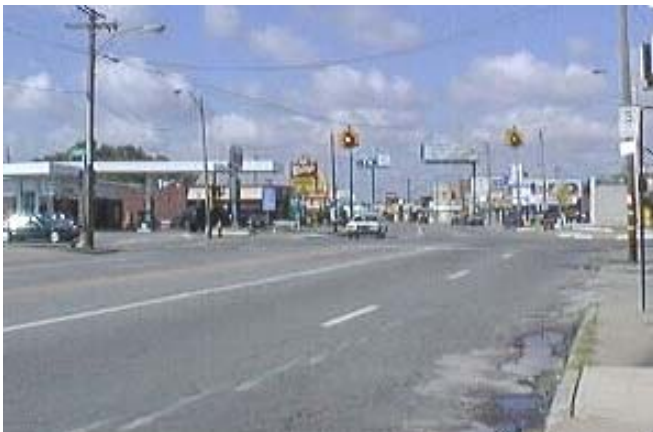
Photograph 25. Eastbound Harper Avenue at Cadieux Avenue ('Before' Condition)
