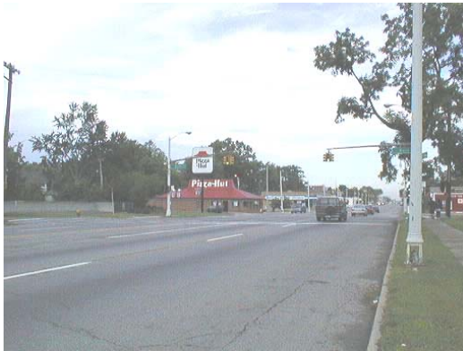
Photograph 5. Grand River Avenue at Burt Road ('Before' Condition)
