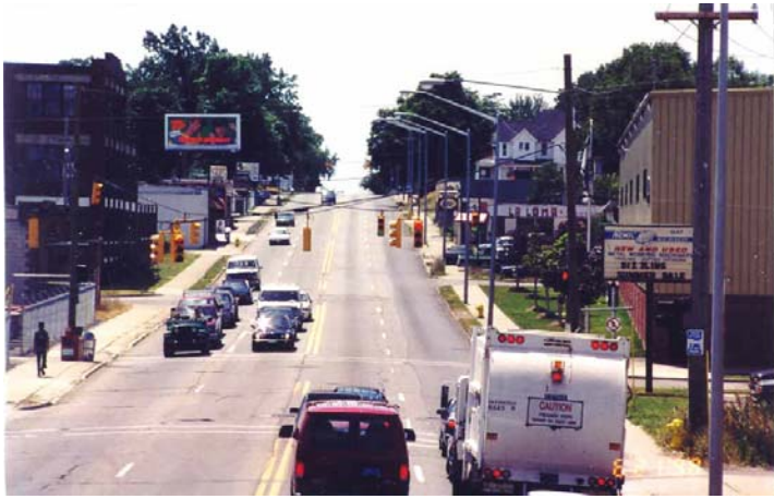
Photograph 23. Division Avenue and Cottage Grove ('Before' Condition)
