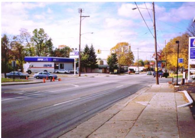
Photograph 15. Westbound Burton Street at Kalamazoo Avenue ('Before' Condition)
