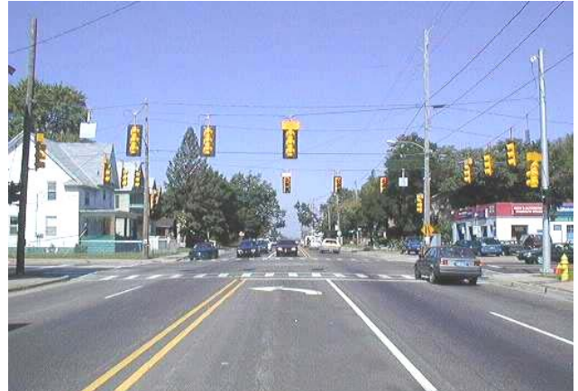
Photograph 14. Westbound Burton Street at Buchanan Avenue ('After' Condition)
