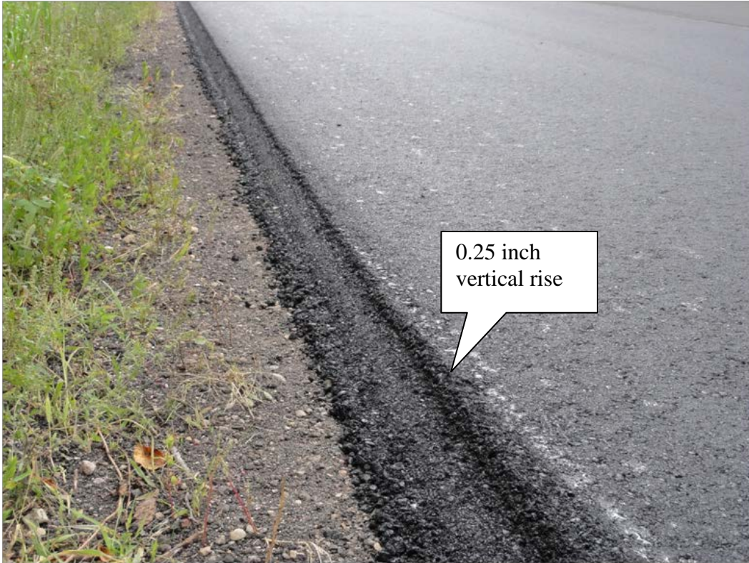
Figure 10. Carlson Prototype #2 edge.
