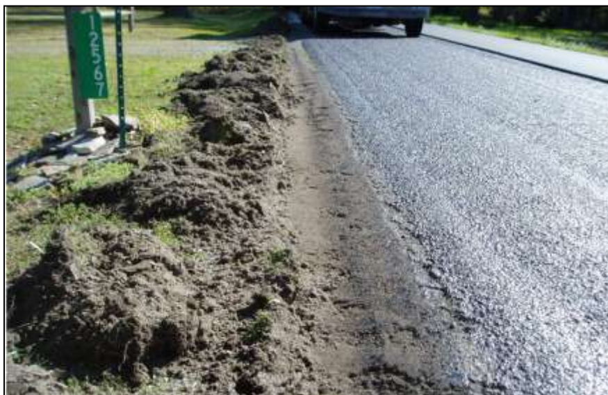
Figure 10. Soil/vegetation piled up from edge preparation work.
