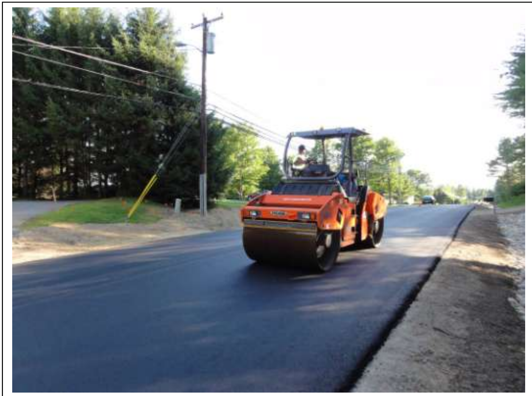
Figure 22. Steel wheel roller used in the finish position.
