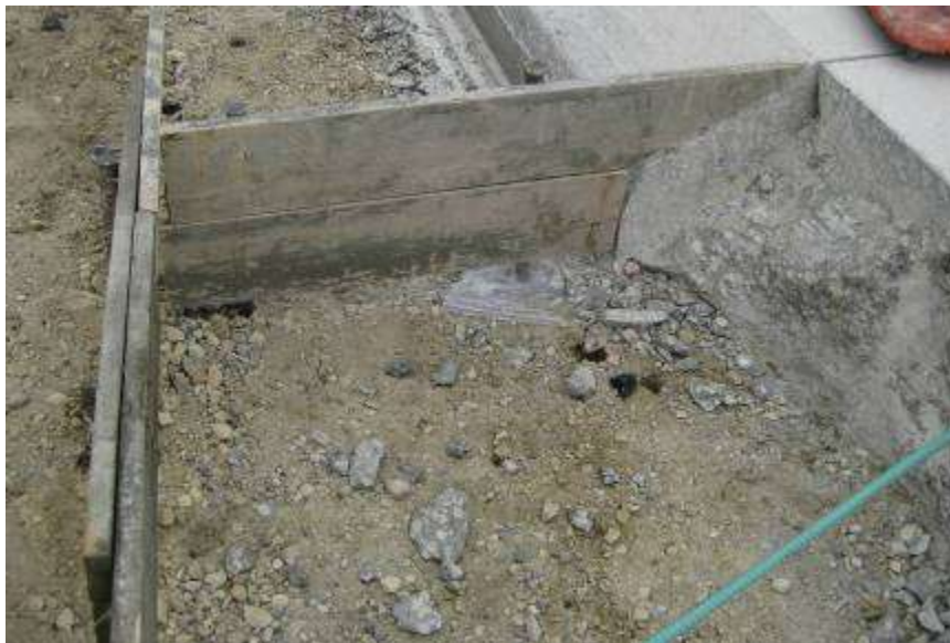
Figure 17. Edge formed and prepared for intersection paving.
