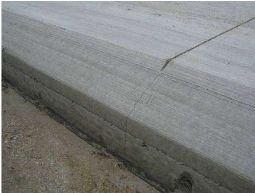
Figure 18: Photo of saw cut and formed joint.
