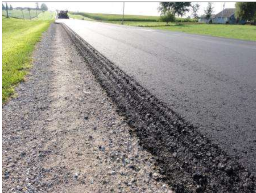
Figure 13. Offset HMA layers with Safety Edges SM .
