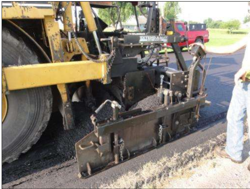
Figure 11. Blaw-Knox paver with the Caterpillar screed.
