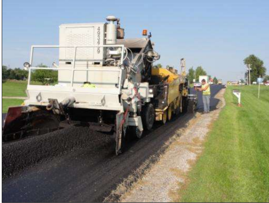
Figure 10. Material transfer vehicle ahead of the paver.
