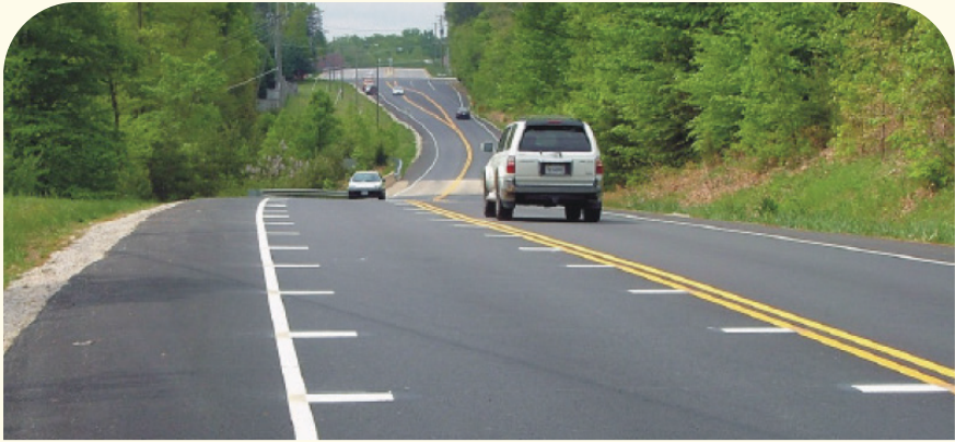
Optical speed bars can increase perceived speed and reduce travel speed. ©Virginia Center for Transportation Innovation and Research.
