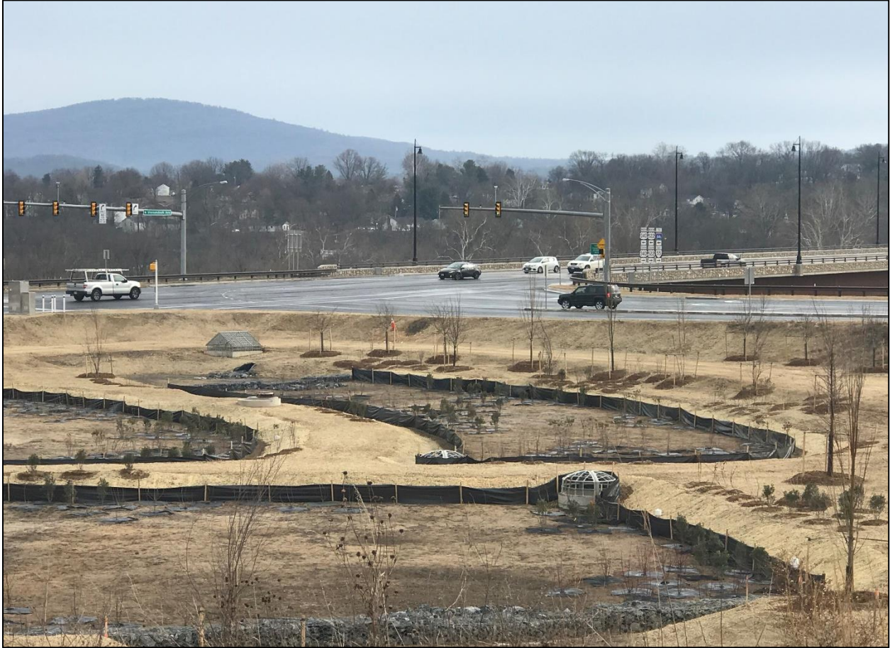
Figure 85. Photo. Use of parcel inside quadrant roadway for bioretention pond.
