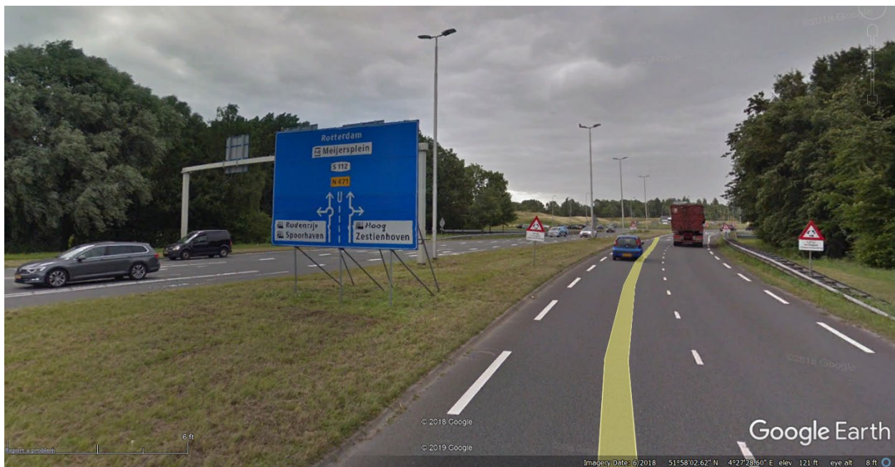
Figure 19. Photograph. Example of guide signage to be placed upstream of a turbo roundabout.
