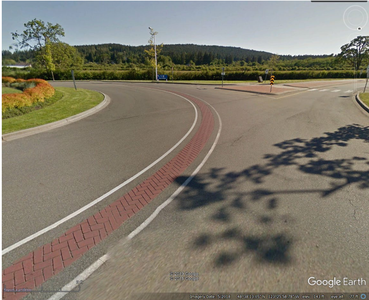
Figure 17. Photograph. Lane divider for turbo roundabout at Victoria International Airport.
