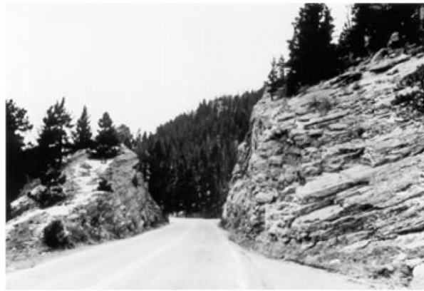
Typical Roadway with Roadside Hazard Rating Equal to 7.
