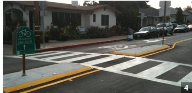
Marked crosswalk with refuge island
