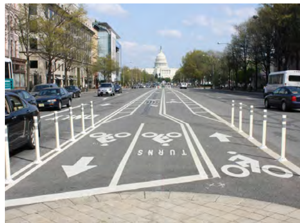
Figure 15. Pennsylvania Avenue bike lanes in Washington D.C. (Photo by Elvert Barnes from pedbikeimages.org)
