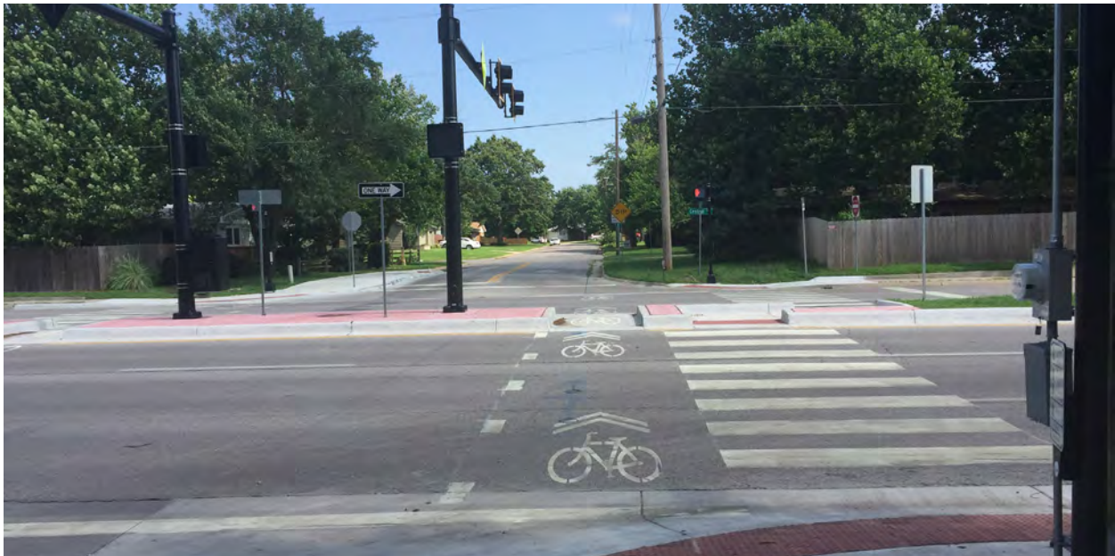
Figure 17. The chapter header image on this page and the photo above show projects shortly after implementation in Wichita, KS. The chapter header image shows a new bike lane and bike box on Market Street. The image above shows a diverter on Woodchuck Boulevard bicycle boulevard to allow for bicycle access. The new pedestrian hybrid beacons help people on foot cross a busy arterial street.
