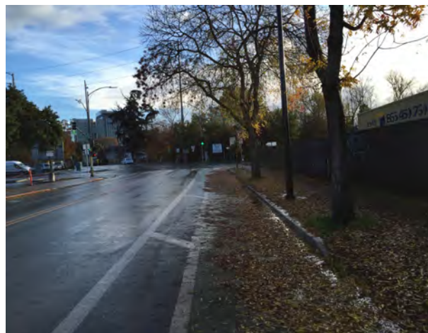
Figure 12. The buffered bike lane pictured above would benefit from street sweeping. Operations and maintenance policies should specify that crews sweep streets from curb to curb, including bike lanes. Special equipment may be needed to adequately maintain barrier separated bike lanes.
