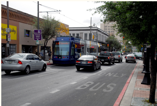
Above: Bus only lane along East Congress Street uses broken lane markings with "Bus Only" and red curbpaint as opposed to the hatched pavement markings found along North 6th Avenue (Photo credit: Dan Nabors).
