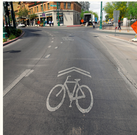
Example of a shared-lane marking placed in the center of the lane (Photo credit: Dan Nabors).
