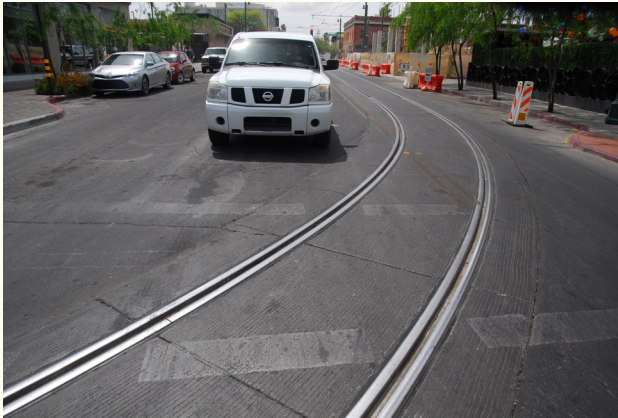
Left turn lane stop bar currently crosses the streetcar tracks, blocking the streetcar if vehicles are pulled forward (Photo credit: Dan Nabors).
