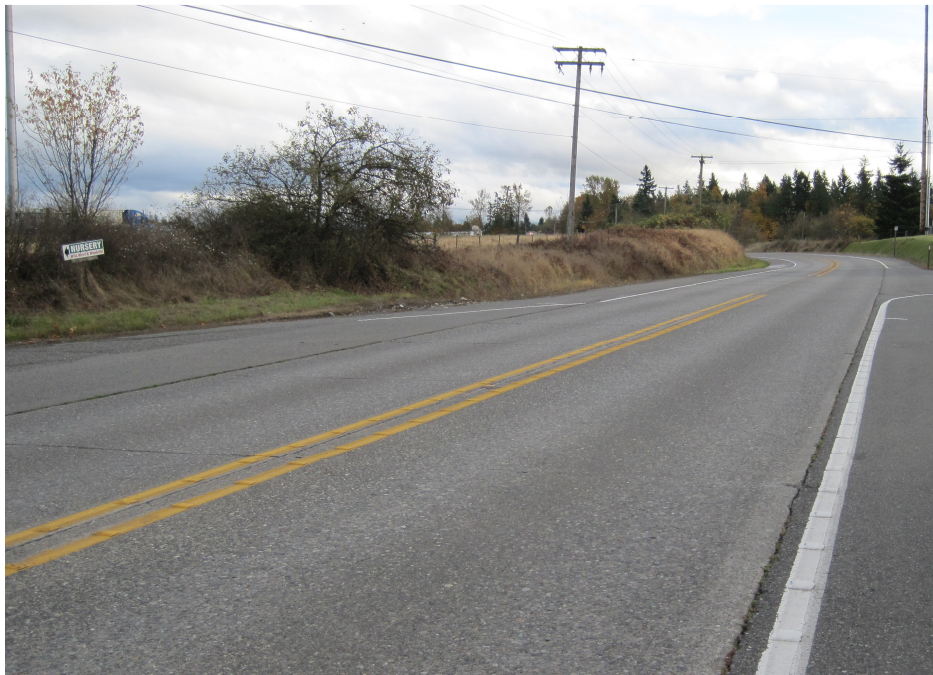
Figure 2. Photograph. Example profiled thermoplastic pavement marking.
