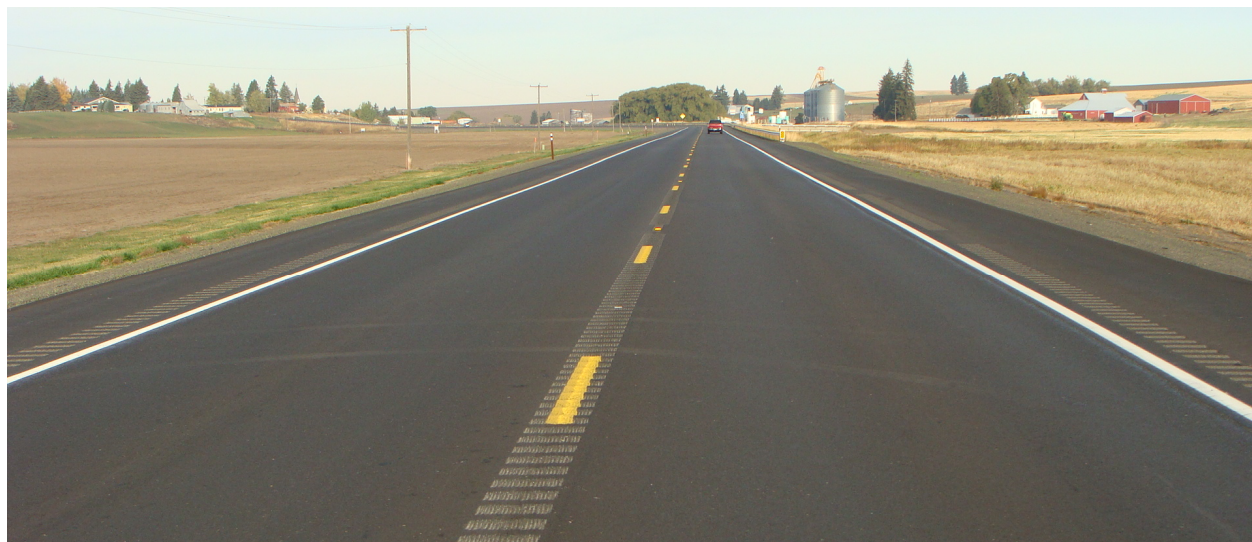
Figure 1. Photograph. Combination milled CLRS and SRS.
