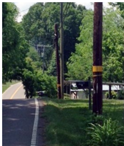
Figure 5. Photo. Yellow prismatic obstacle delineation around a roadside pole in Tennessee.
