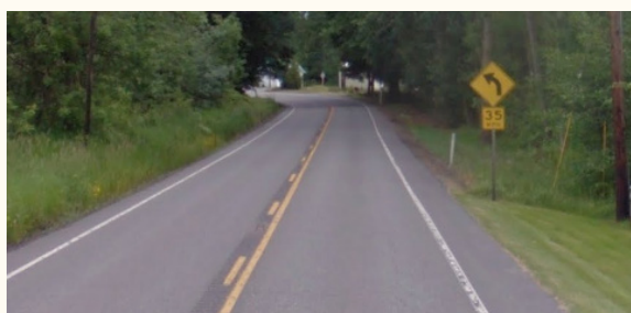
Top: Southbound view of the curve at the intersection of SR 7, Tanwax Road, and 66th Avenue. This curve is fairly flat, particularly in comparison to the curve to the south. Bottom: Southbound view of northern curve, at the intersection of SR 7, Tanwax Road, and 66th Avenue. This curve warning sign is the only one used on the curve in either direction. There are also a couple post-mounted delineators. (Credit: Dan Nabors)
