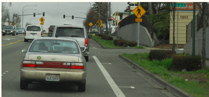
Near the intersection of SR 7 and 116th Street, there are several intersections and driveways with limited sight distance due to the retaining walls and change in elevation. The limited sight distance increases the risk in this location, where there are numerous conflict points as drivers turning left from side streets or driveways cross sidewalks, bike lanes, four travel lanes, and a two-way left-turn lane. (Credit: Dan Nabors)
