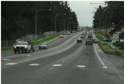
SR 7 near the intersection at 159th street: a wide edgeline separates the vehicular travel lanes from the bike lanes. The edge lines are not present or are much narrower on the northern portion of the corridor. (Credit: Dan Nabors)
